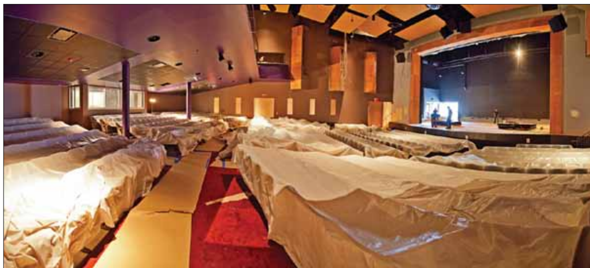
Interior of the Performing Arts Center during the final stages of construction in June.
